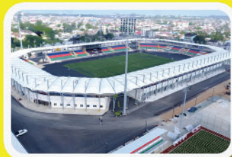
CONSTRUCTION OF SPORTS FIELDS
