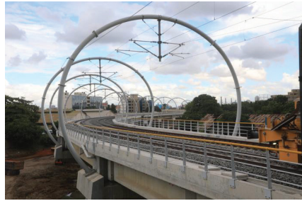
SGR infrastructure in Dar es salaam
